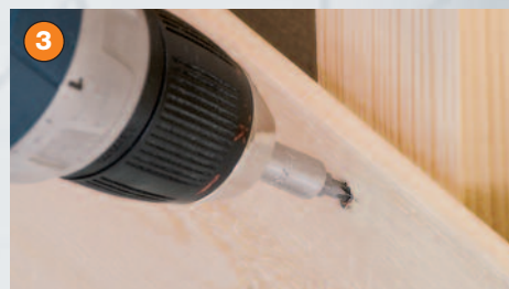
3 Gap free axial fixing of the timber board via the HECO-UNIX full thread
