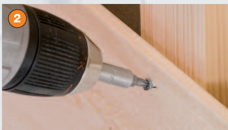
2 The smaller thread pitch means that the boards are clamped firmly together
